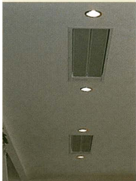
An additional aluminium frame encases EnergoStrip, allowing flush-fixing into a solid or gibbed ceiling.
