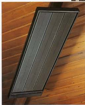
EnergoStrip heaters installed in St Michael's Anglican Church, Christchurch. The satin-black finish is an optional extra.
